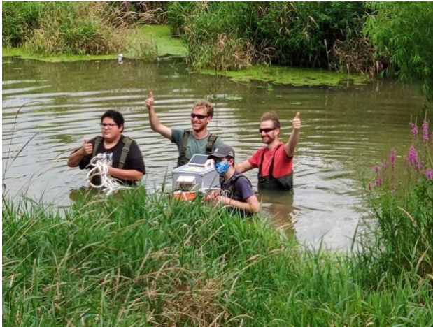
Figure 3: Installing sensors in McKenzie Creek.
