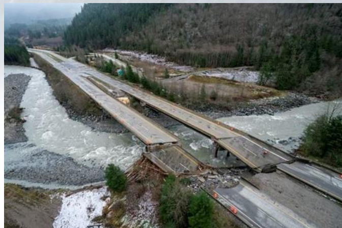
The Coquihalla Highway near Hope, British Columbia was severed by floodwaters and debris flow resulting from record-setting heavy rainfall in November, 2021. It was found that human-caused climate warming increased the probability of this event by roughly 50% (see https://doi.org/10.1016/j.wace.2022.100441 ).
