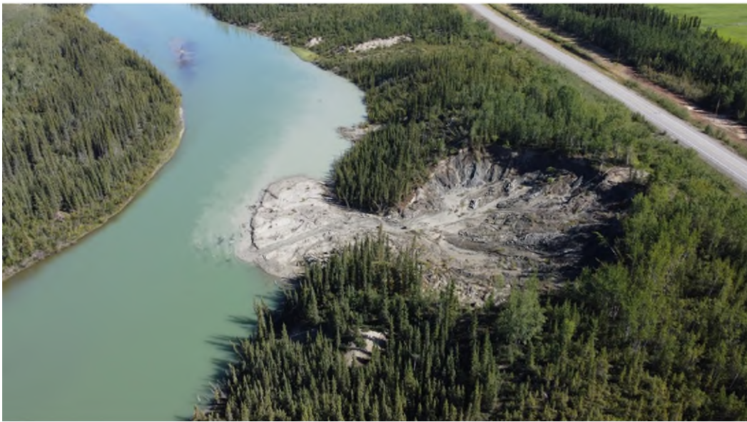
Permafrost slump near highway in Yukon. Photo by Mark Ferguson
