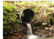
Culvert Assessment and Flood Modelling in Rural Saskatchewan
