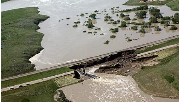
Highway 01, Culvert Crossing Near Maple Creek, SK Flood Event 2010
