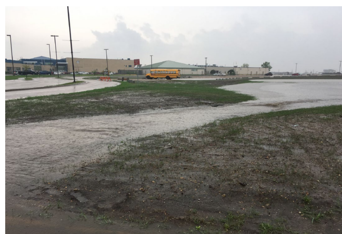
Flooding in Humboldt, 2018.
